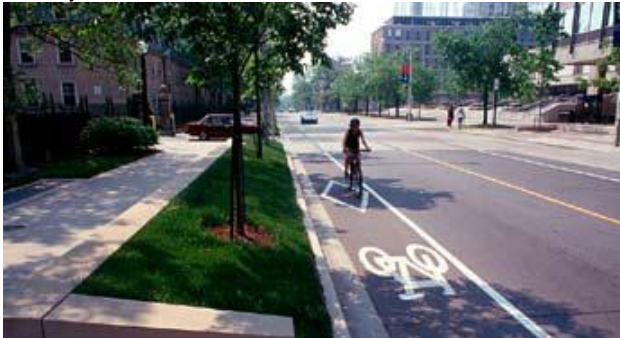
Lane reduction from two to one lane in each direction, bike lanes, and center turn lane.
