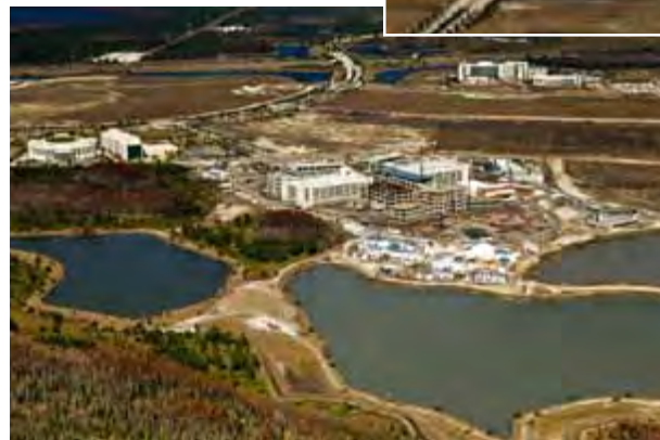
Aerial views of Orlando Medical City under construction in Lake Nona.
